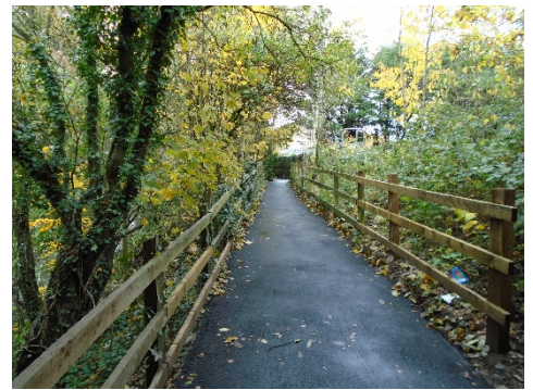
New footpath surface near Lanelay Park
